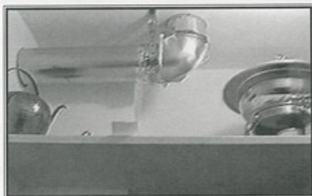
Proper duct joints should be connected with heat resistant tape.
